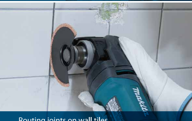
Routing joints on wall tiles
