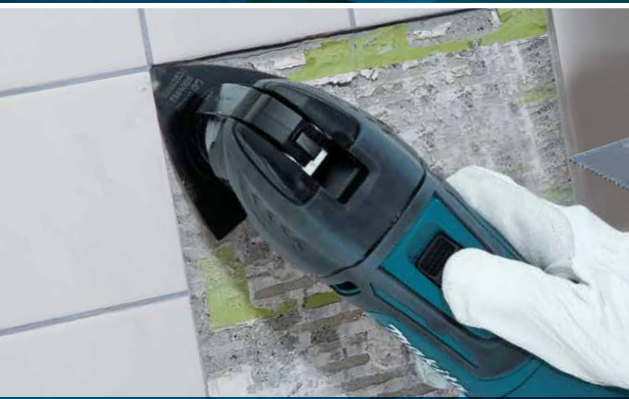
Removing mortar, tile adhesive
