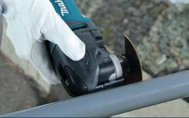
Cutting PVC, FRP pipes
