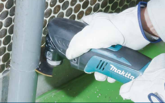
Cutting PVC, FRP pipes
