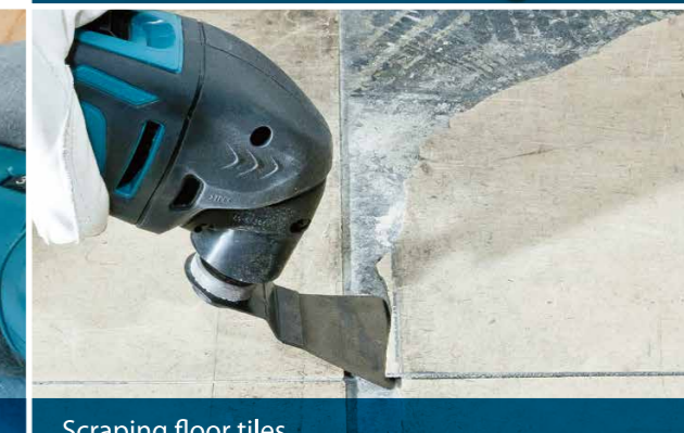
Scraping floor tiles
