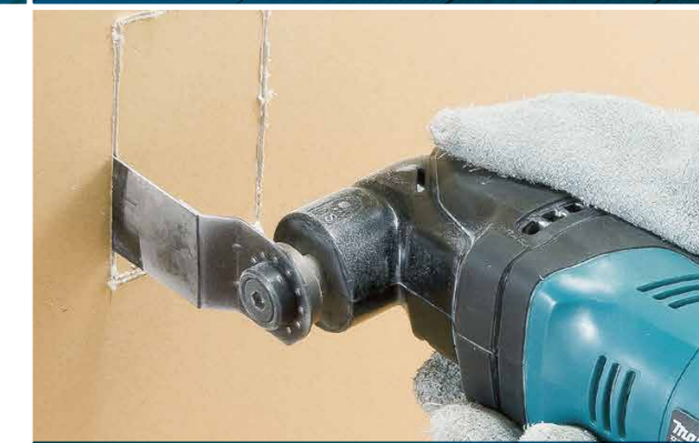
Cutting plasterboards
