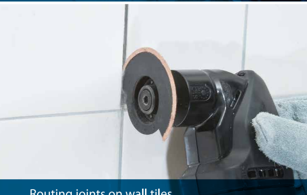
Routing joints on wall tiles
