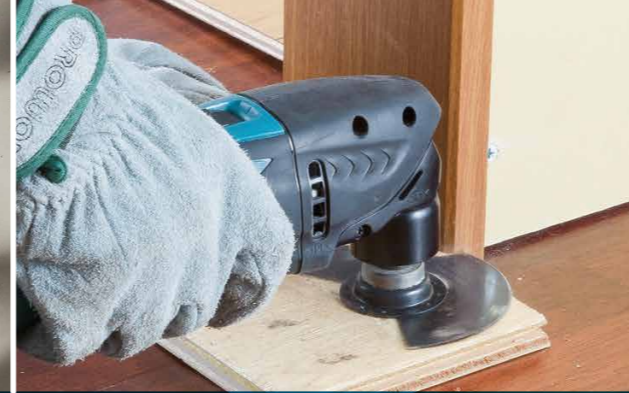
Wood flush cutting
