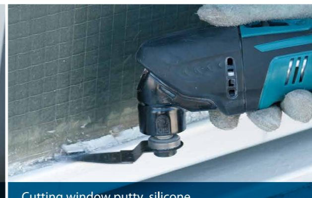
Cutting window putty, silicone
