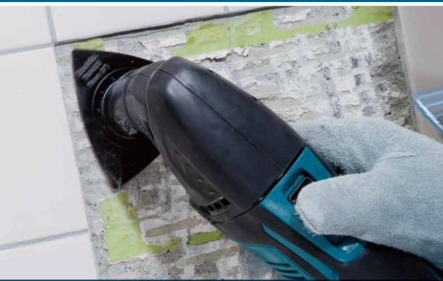
Removing mortar, tile adhesive
